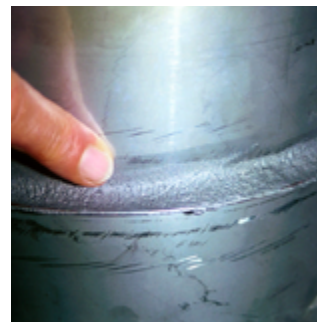
Pyro-Putty® 2400 seals high temp ducting.
