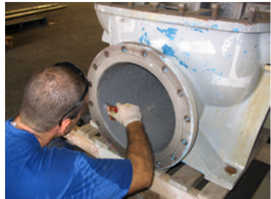
Corr-Paint™ CP2060 coats pump housing.
