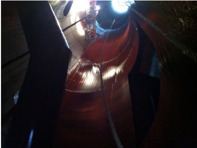
Corr-Paint™ CP2050-LF coats flare stack.
