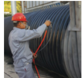
HiE-Coat™ 840-M coats industrial heat exchanger.
